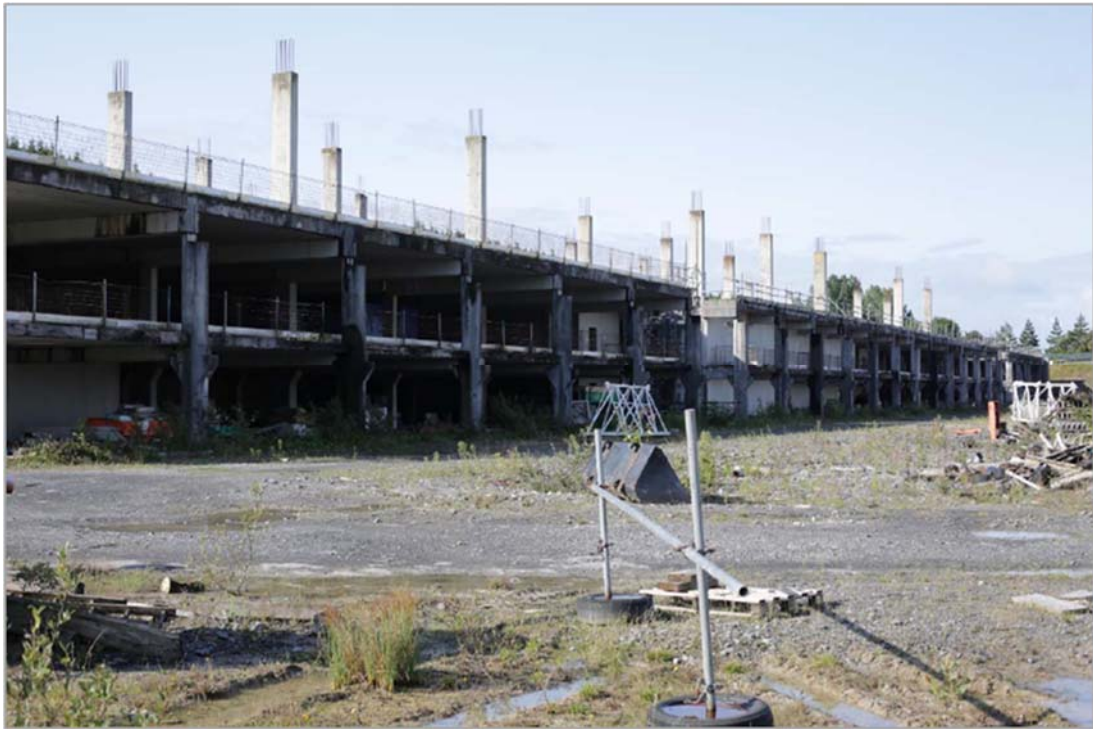
Plate 2: Internal view of the site towards the partially constructed double basement car park located along the South-Eastern site boundary
