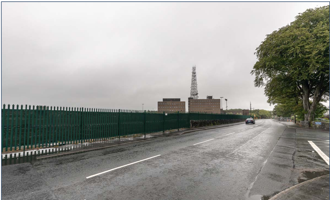
Plate 6: View from Monivea Road at junction with Clark Avenue looking North-East towards the proposed site
